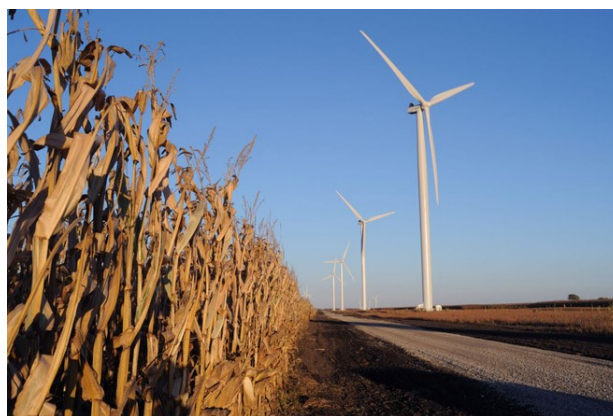
Meadow Lake wind farm Source: EDP Renewables
