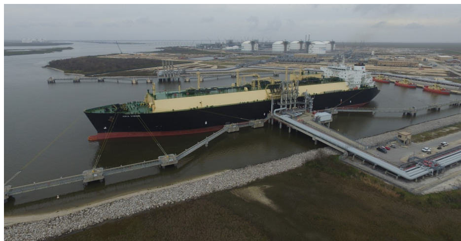
Loading of the first cargo at the Sabine Pass LNG Terminal in February 2016. Source: Cheniere
