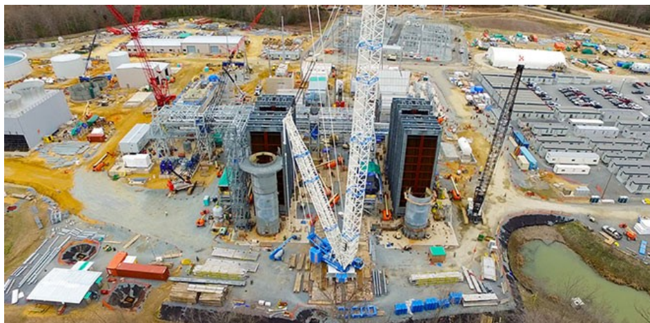
CPV St. Charles under construction in January 2016 Source: Competitive Power Ventures
